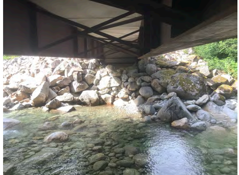
Left Bank Abutment when facing downstream
