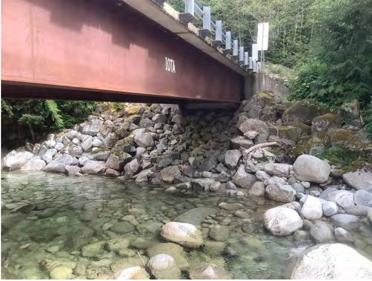
Right Bank Abutment when facing downstream
